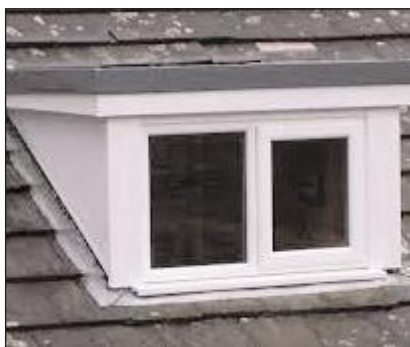
A dormer roof similar to the one Lisa was having repaired
